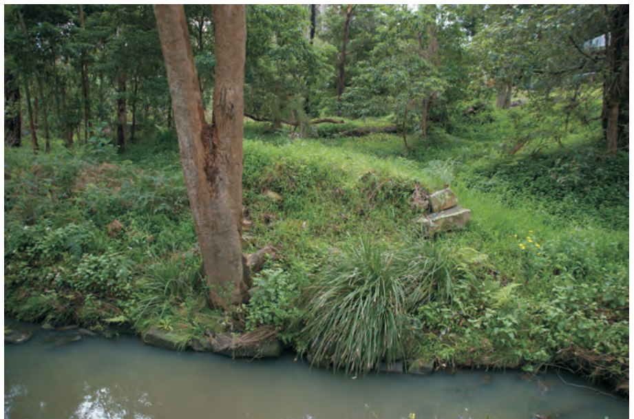
Figure 3: Tree in northern abutment has displaced a large amount of stone from the abutment. This tree is the highest priority for removal if the stonework is to be conserved.
