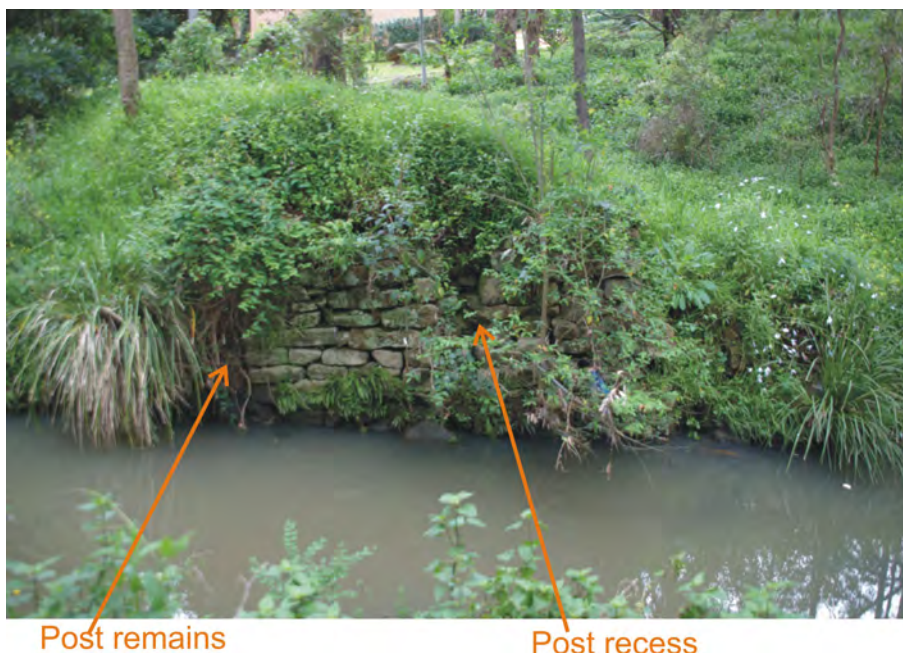
Figure 1: Southern abutment with arrows showing the post locations.
