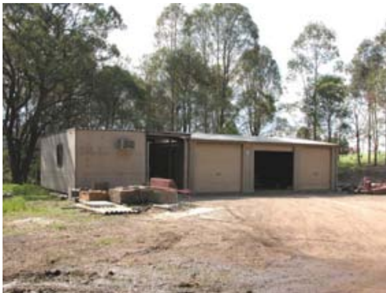
Fagan Park works depot. These temporary buildings require upgrading to provide better staff facilities and improved security for equipment. (Photo: C Betteridge, 24 April 2003)
