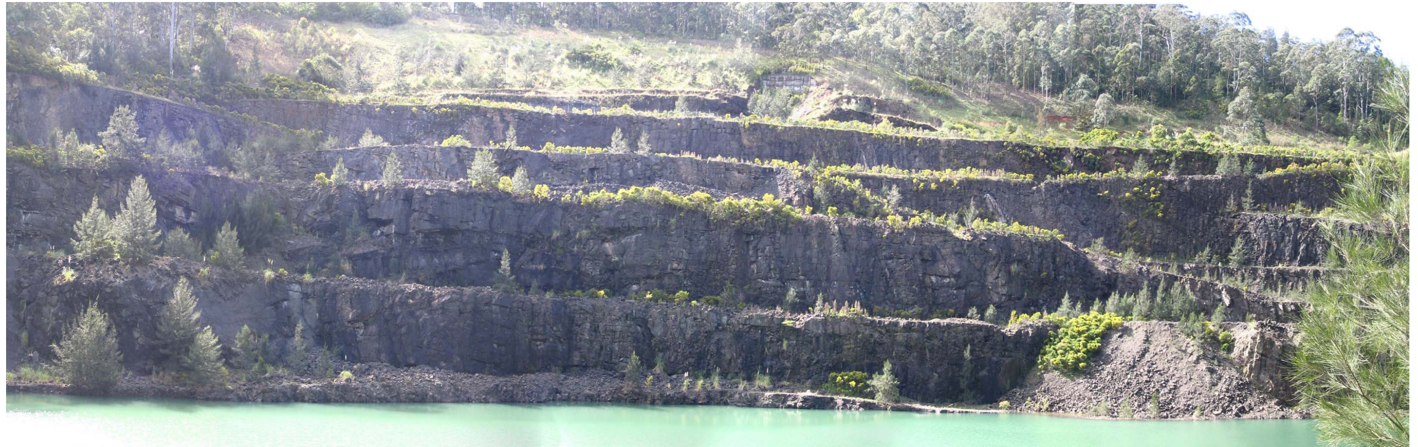
Plate 1: Lower North Wall of Hornsby Quarry
