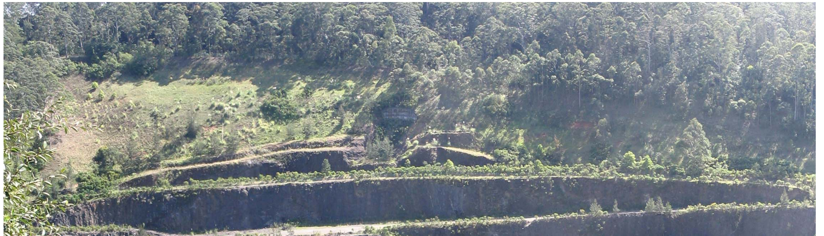
Plate 2: Upper North Wall of Quarry
