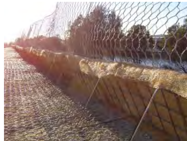
Green Terramesh units with pre-formed angle & Biomac
