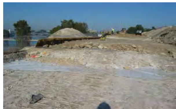
Rock PEC geotextile composite basal reinforcement
