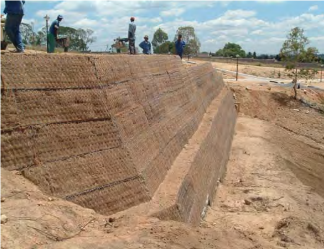
2005. East London, South Africa. Green Terramesh™ reinforced slope. Photos were taken during installation.
