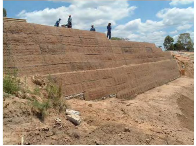
2005. East London, South Africa. Green Terramesh™ reinforced slope. Photos were taken during installation.
