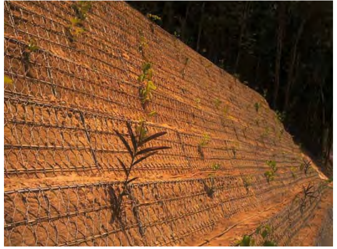
2005. Kuranda Range, Cairns. 36m long x 5.4m high Green Terramesh™ reinforced slope. Photos were taken soon after installation.
