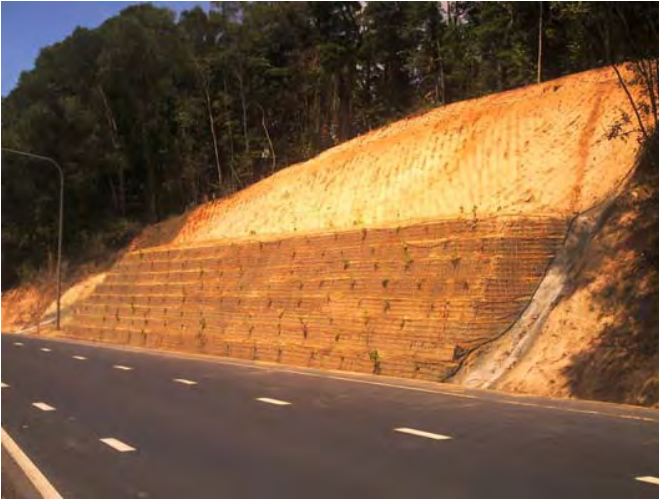
2005. Kuranda Range, Cairns. 36m long x 5.4m high Green Terramesh™ reinforced slope. Photos were taken soon after installation.
