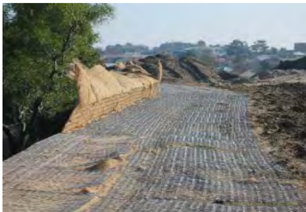
Green Terramesh integral tails (pre-determined lengths)
