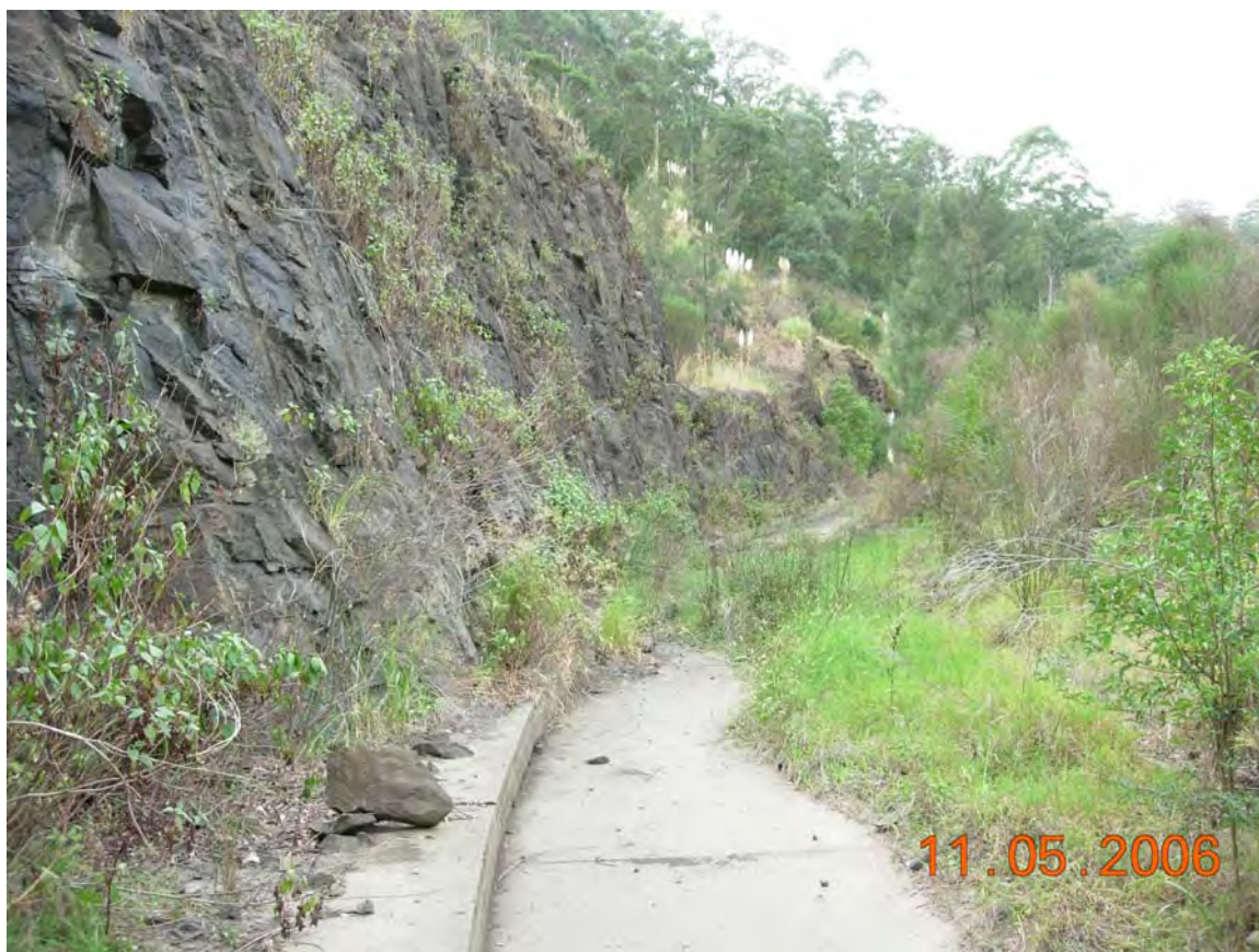
Photo F4: Existing Diversion Channel
