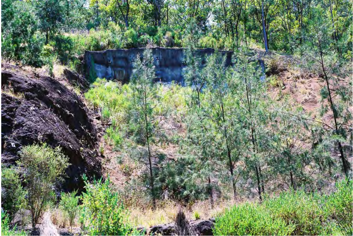
Photo F8: Existing Stabilisation Works in Old Slip Area above Proposed Walking Track at about Chainage 180m (see Figure F1)
