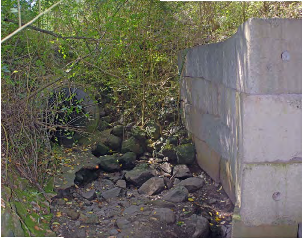
Photo F7: Pipe Outlet
