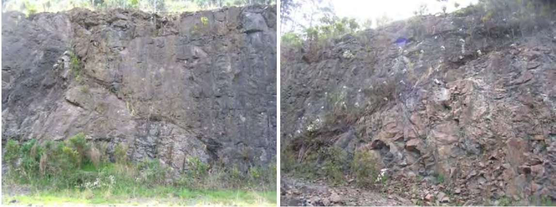
Photo A4: Two examples of sheared zones in Hornsby Quarry
