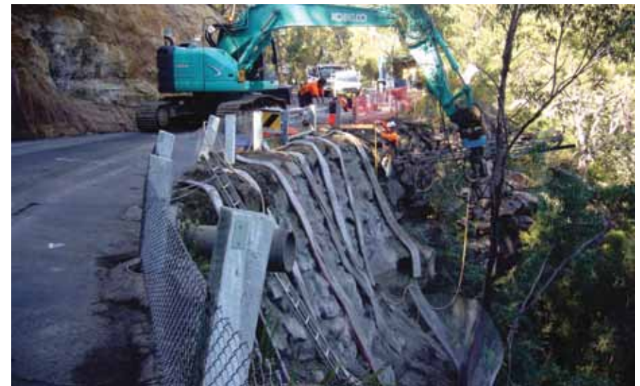
Berowra Waters Road work
