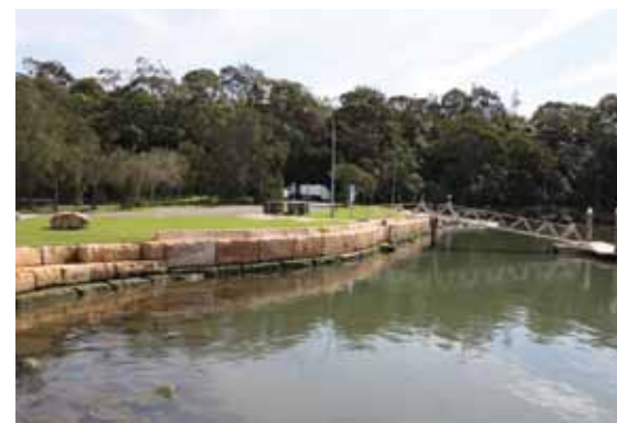
New seawall, Parsley Bay, Brooklyn
