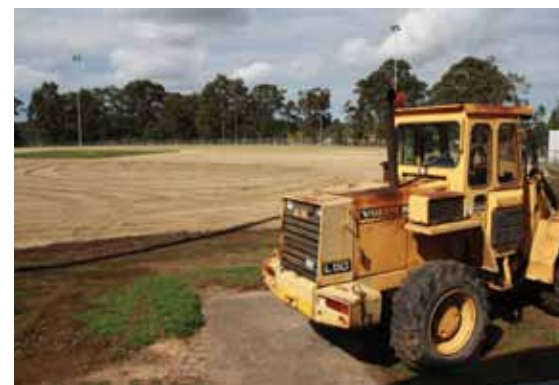
Drainage upgrade works – North Epping Oval
