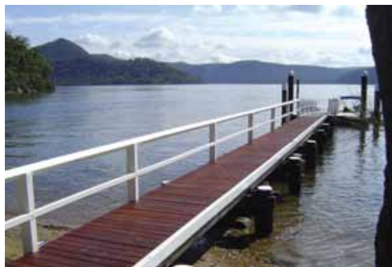
The new Bar Island Jetty
