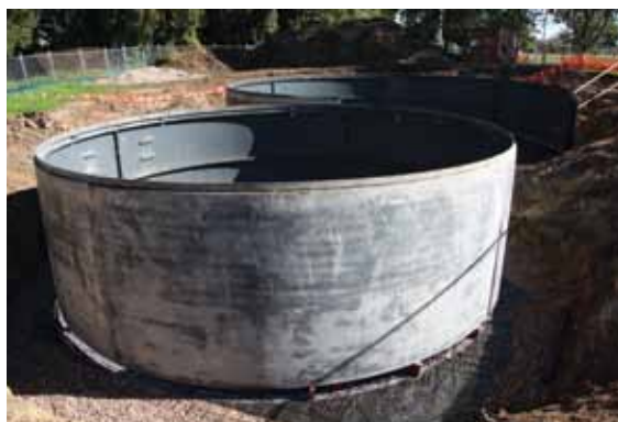
Underground stormwater tanks, Epping Oval
