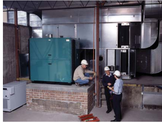
Construction of Cogeneration System at Hornsby Central Library
