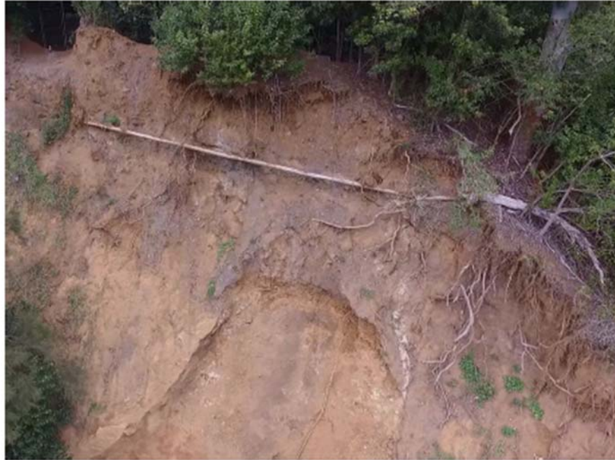
Plate 12. View of recent slide in extremely weathered rock at crest of south wall.
