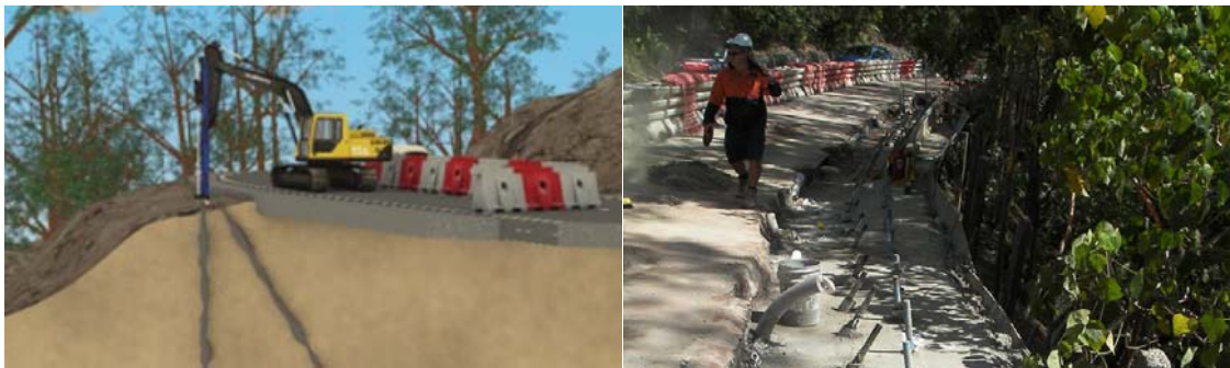
Figure 51 Illustration of micropile installation process and photograph of partially completed micropile wall
