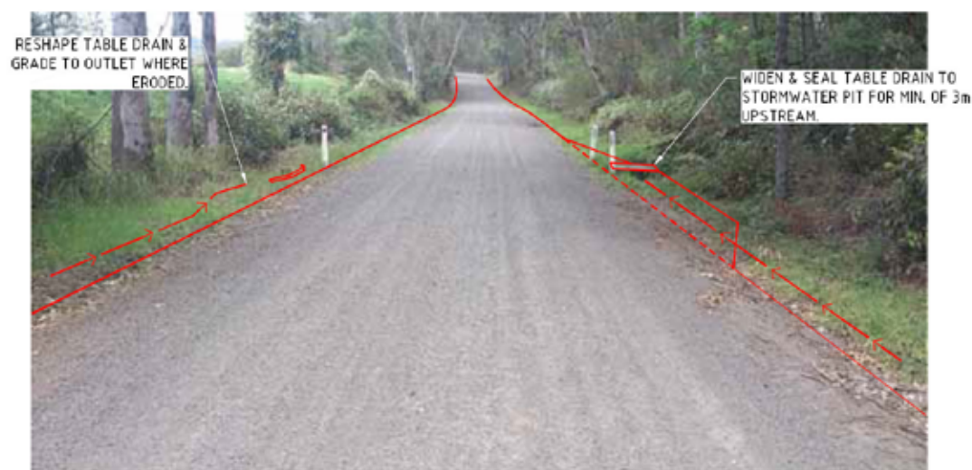
MID-SECTION TYPICAL MAINTENANCE OF PIPE CROSSINGS
