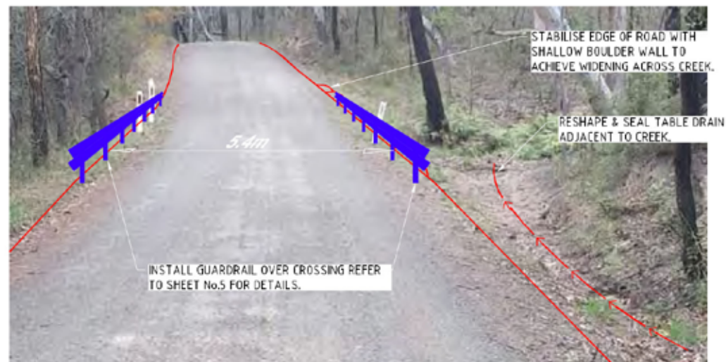
CULVERT CROSSING AT CH730.00 MAINTENANCE OF EXISTING CREEK CROSSING
