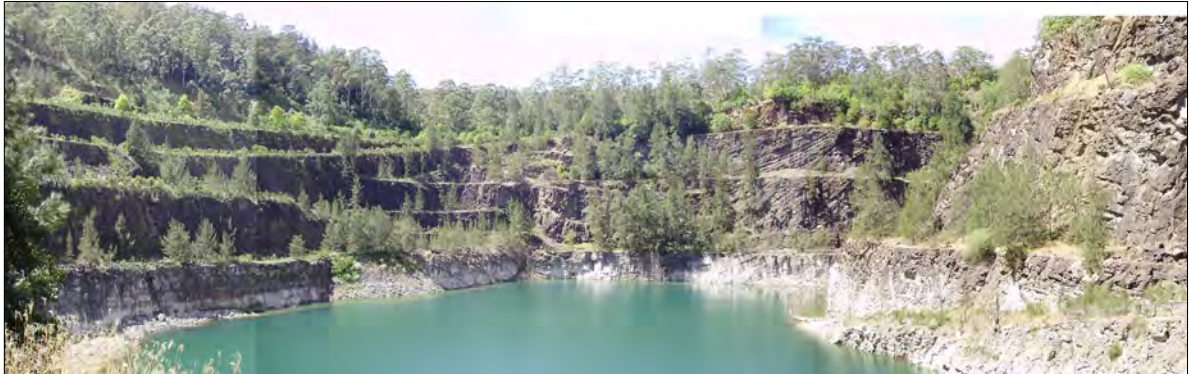
Hornsby Quarry - view from western side of quarry, looking east showing diatreme
