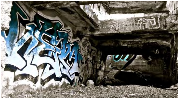
Old quarry buildings and structures
