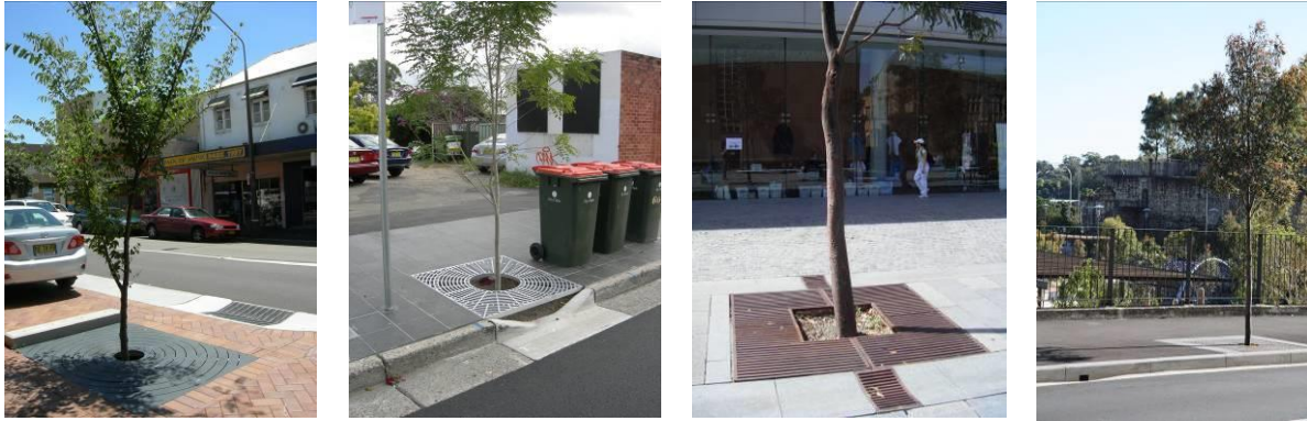
Figure 2: WSUD in Street Tree pits - Hornsby (left), Meadowbank shops, Ryde (centre left), Sydney University (centre right) and Pirrama Park, City of Sydney (right) (Photos: Equatica).
