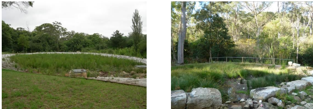
Figure 3: WSUD rain-gardens in in Hornsby LGA – Lyne Road, Cheltenham (left), Oorin Road, Hornsby Heights (right) (Photos: Equatica).
