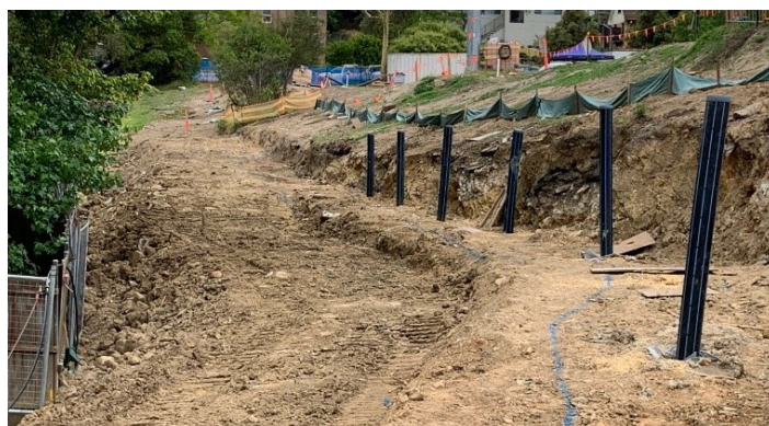
Figure 1: Installation of the below ground bores along the northern batter
