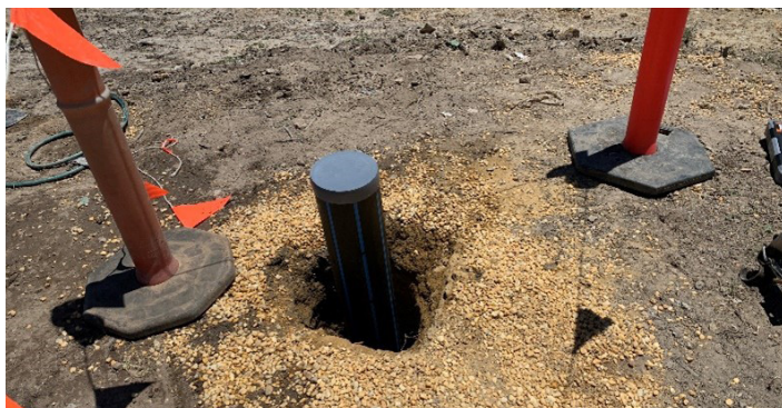
Figure 2: Capped underground bores which will be connected to the underground gas feeder pipes.
