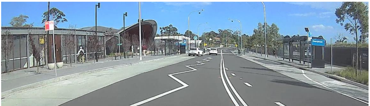
Figure 3-69: Bus station on Bradfield Road
