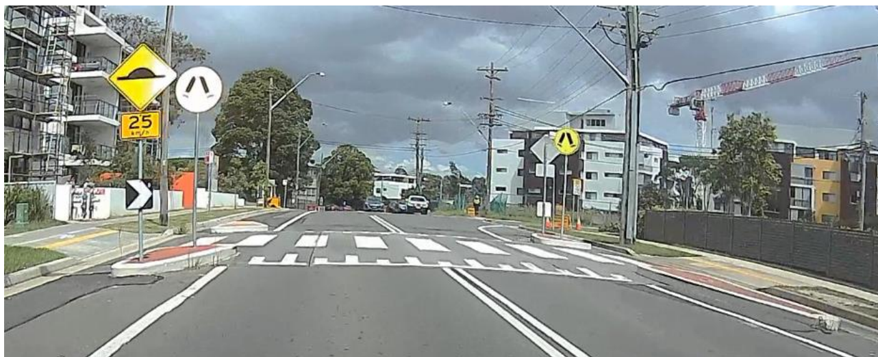
Figure 3-25: Raised pedestrian crossing on Peats Ferry Road
