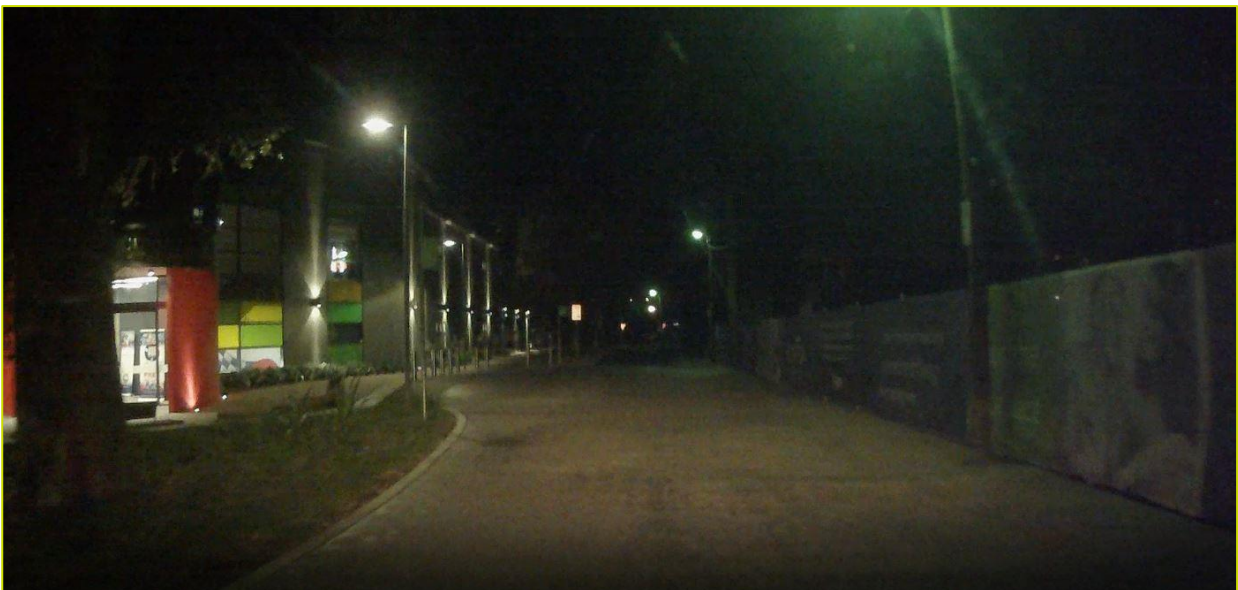
Figure 2-38: Lighting on Park Lane
