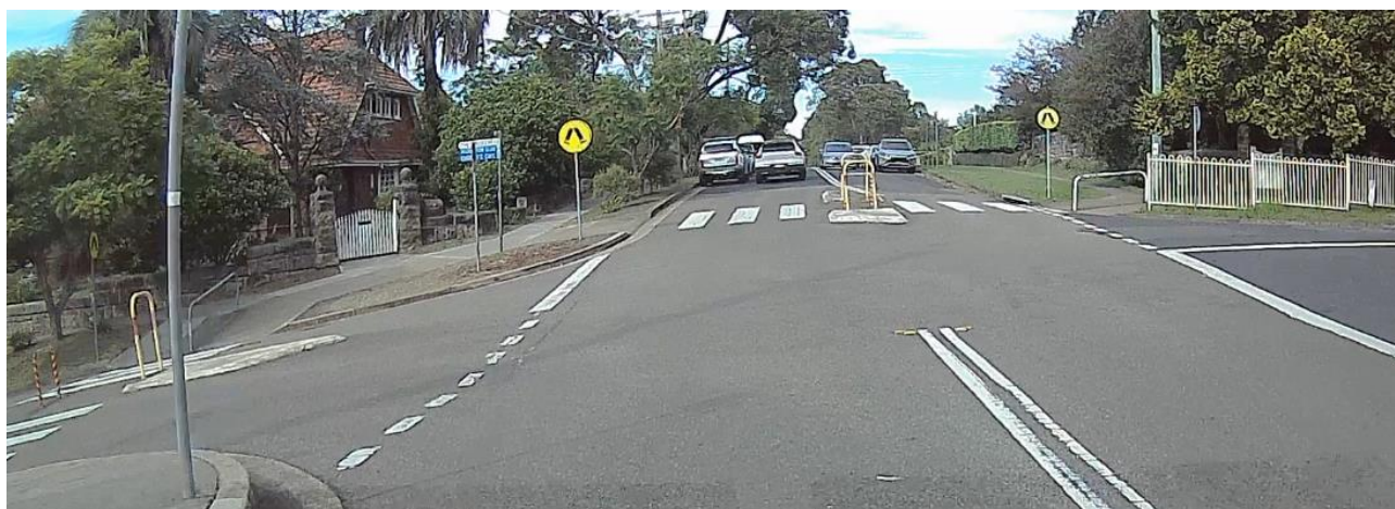
Figure 3-35: Pedestrian crossings at the intersection of The Crescent and Cheltenham Road
