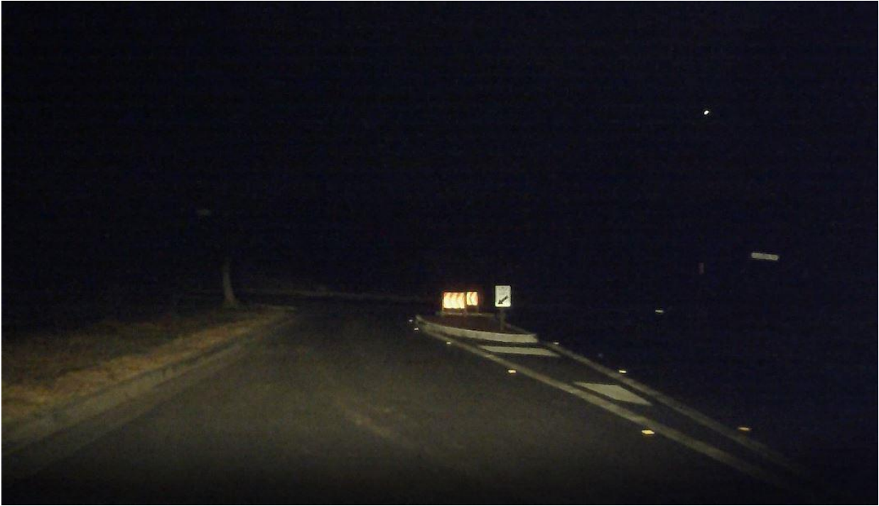
Figure 2-48: No lighting at the pedestrian refuge island on Balmoral Street
