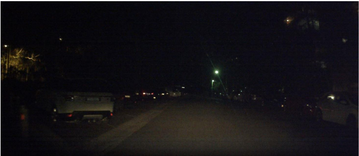
Figure 2-49: Limited street lighting on Leonard Street
