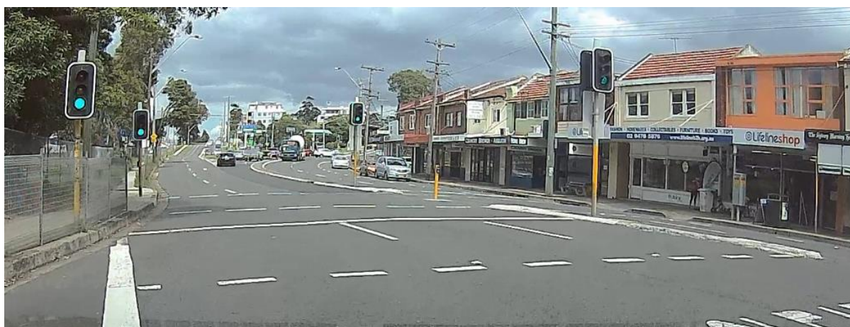
Figure 3-24: Signalised pedestrian crossing on the Pacific Highway
