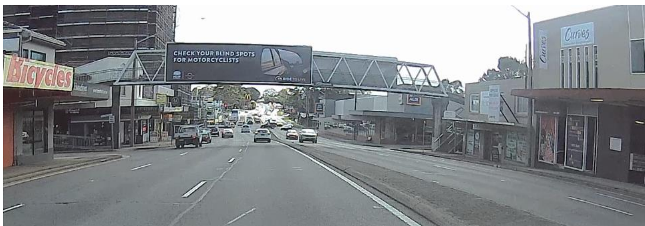
Figure 3-49: Pedestrian overpass across the Pennant Hills Road
