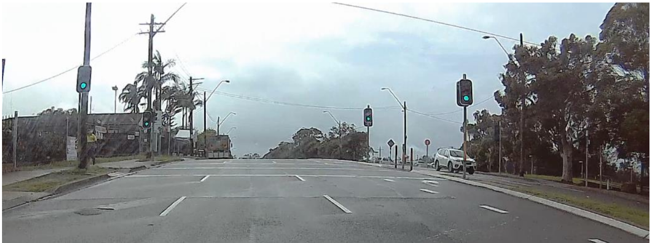
Figure 2-50: Signalised pedestrian crossing on the Pacific Highway
