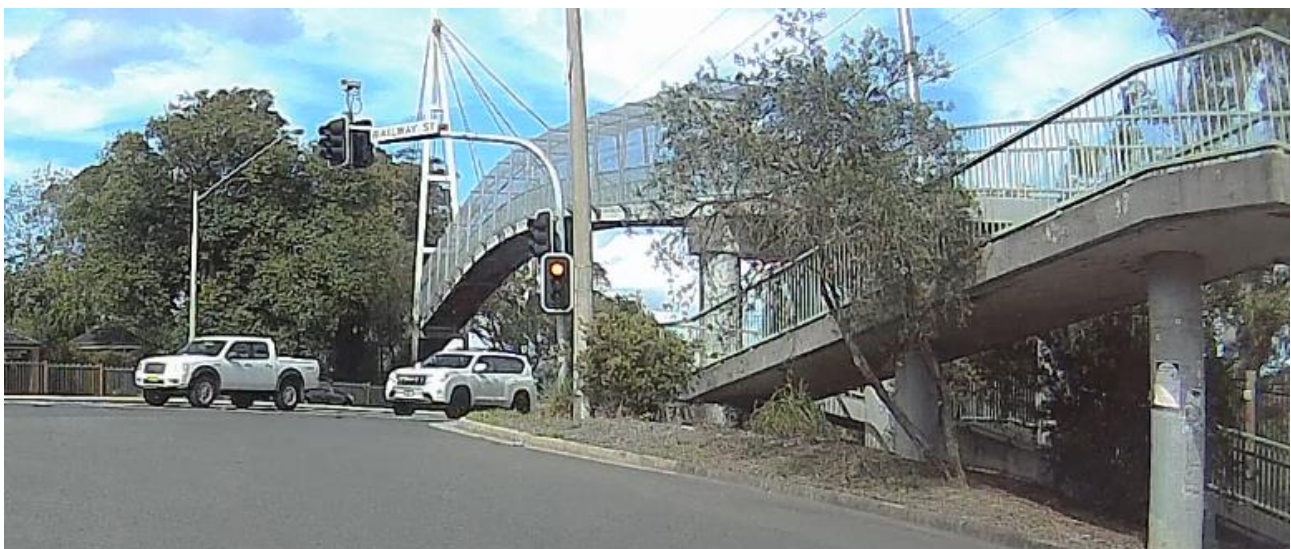
Figure 3-38: Pedestrian overpass across the Cumberland Highway
