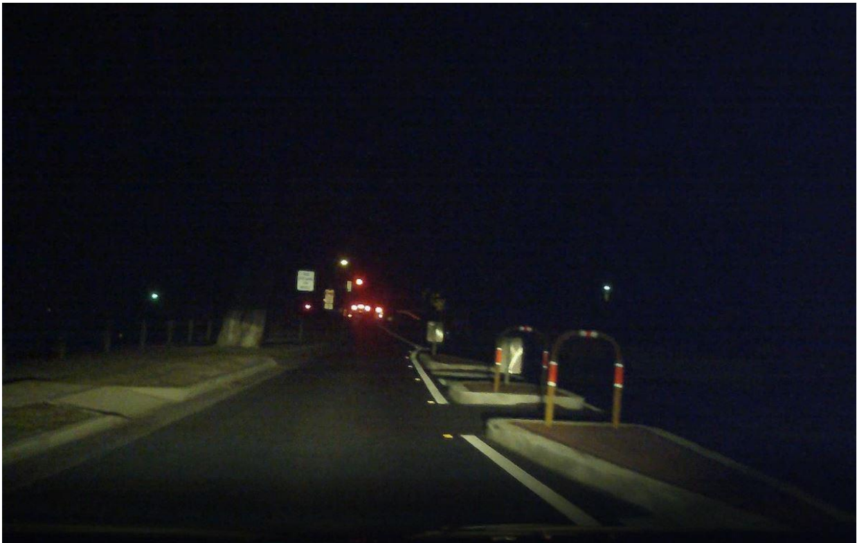
Figure 2-47: No lighting at the pedestrian refuge island on Ingram Road
