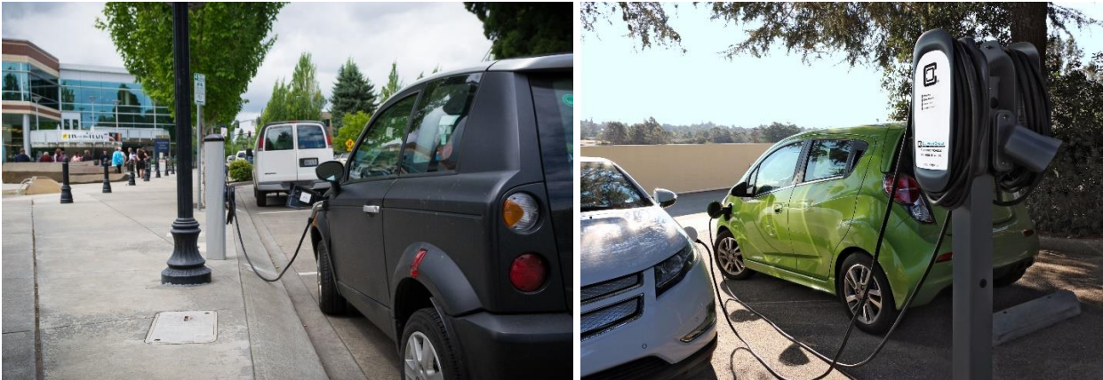
Figure 10.1: Examples of on-street and off-street electric vehicle charging stations
