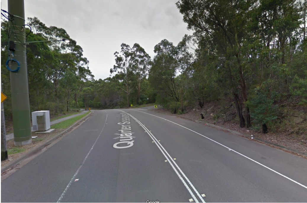
Figure 4 – Existing Intersection Warrigal Drive (southern end) with Quarter Sessions Road – Looking North
