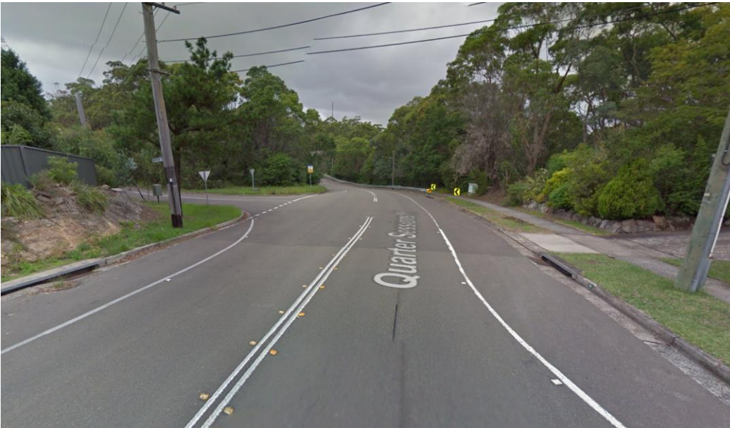
Figure 7 – Existing Intersection Warrigal Drive (Northern End) with Quarter Sessions Road – Looking South
