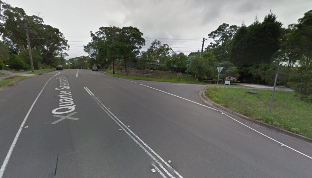
Figure 6 – Existing Intersection Warrigal Drive (Northern End) with Quarter Sessions Road – Looking North
