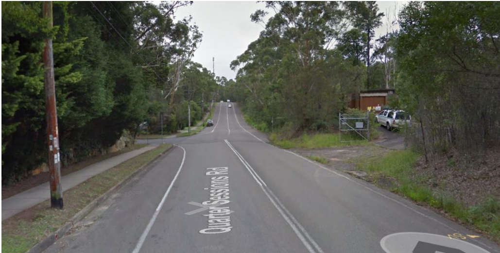
Figure 8 – Existing Southern Access with Quarter Sessions Road near Corang Road – Looking North
