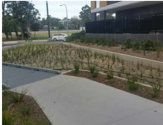
Orara Park, Waitara (for irrigation of Mark Taylor Oval) - biofilter and stormwater harvesting system
