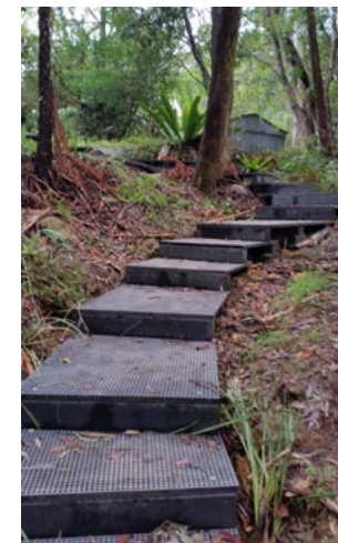
Waitara Creek bushland, Normanhurst - fibre reinforced polymer steps
