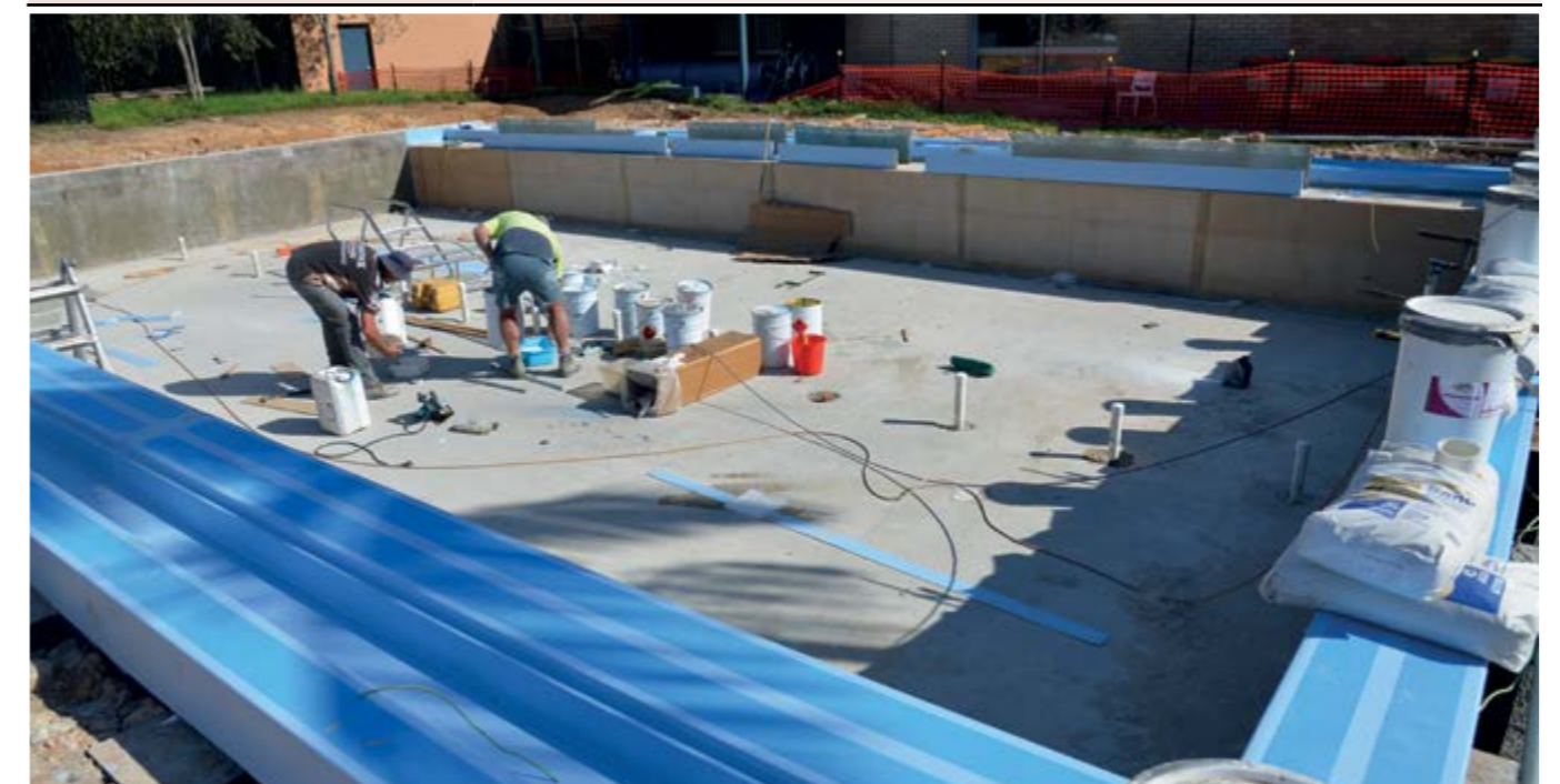
Construction underway of Galston Learn to Swim Pool
