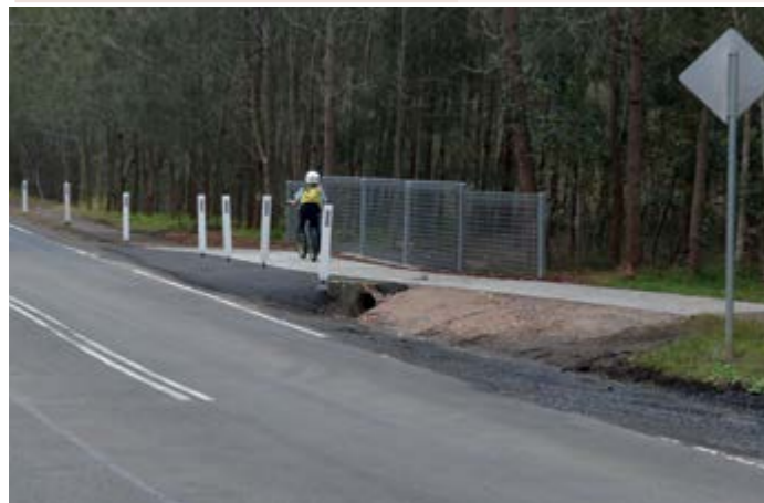
Brooklyn Road, Brooklyn - stormwater drainage culvert
