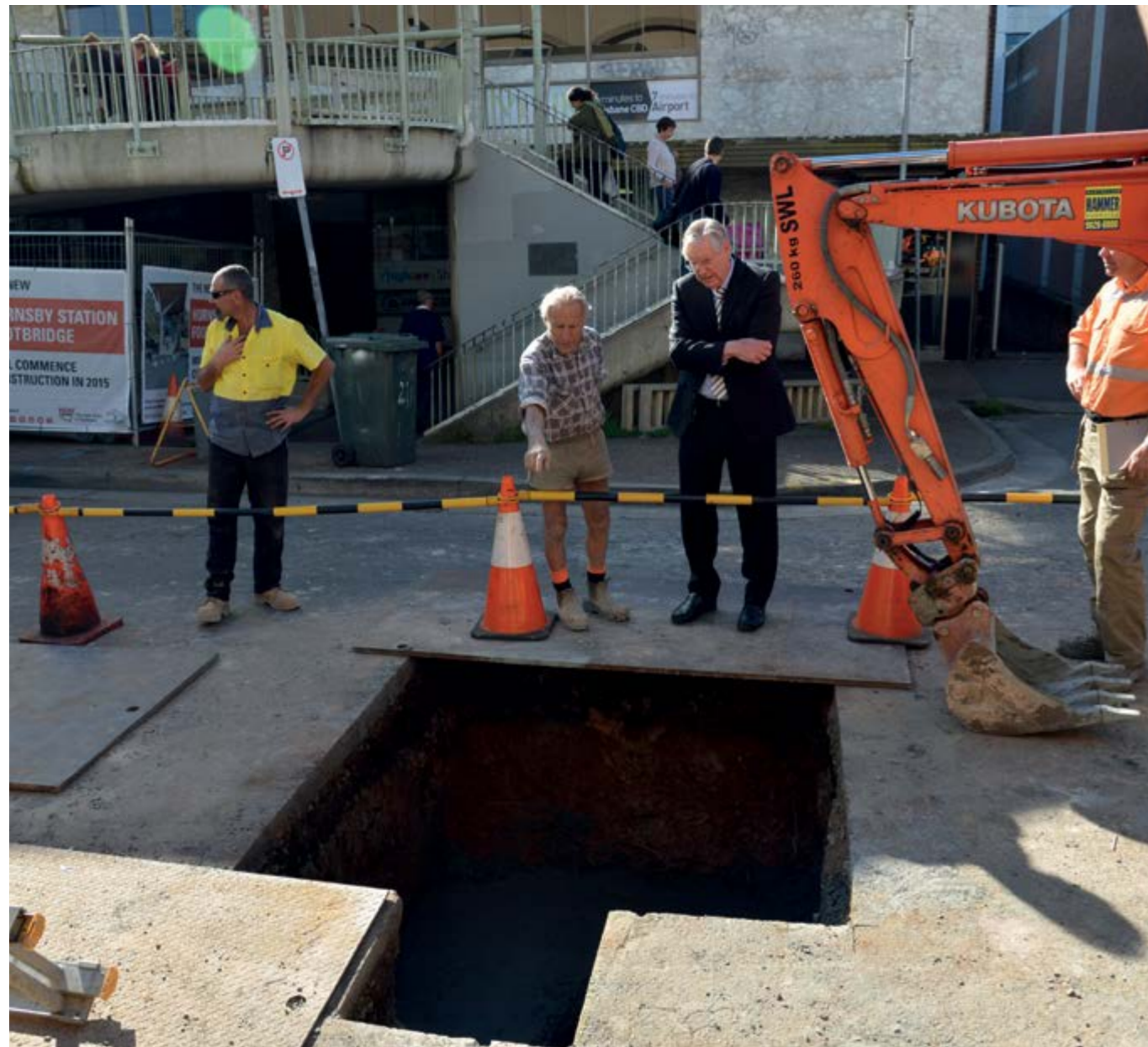
Preparation works for new Hornsby Station Footbridge
