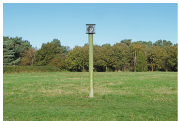
Figure 1: Typical landfill gas vent
