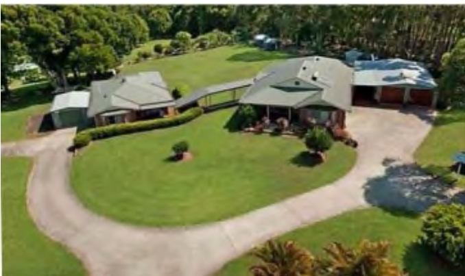
Figure 2.2-b: Covered walkways are not acceptable means of attaching the two dwellings (E)
