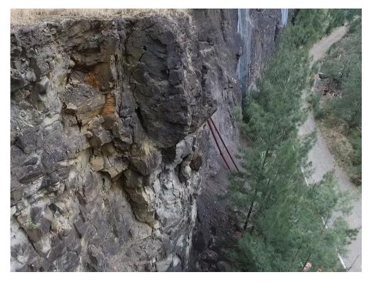
Plate 19. View of loose rock, open joints and mesh along the west wall.
