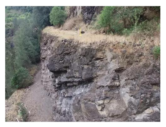
Plate 11. Blast damage and fretting / erosion of breccia horizons at the south-eastern corner of the quarry adjacent to proposed conveyor location. Note: scree material on bench below.
