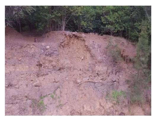
Plate 13. View of recent slide in material mounded at crest of south wall. Note: intact blocks of rock (corestones) exposed in batters.
