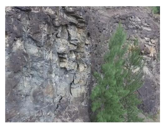
**Plate 10.** Drill holes with adjacent blast damage / open fractures and fretting of muddy breccia horizons at the northeastern corner of the quarry.
