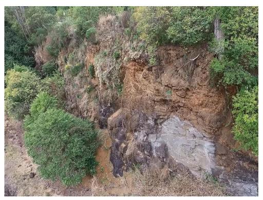
Plate 8. Extremely to highly weathered breccia horizon on uppermost batter of the east wall.
