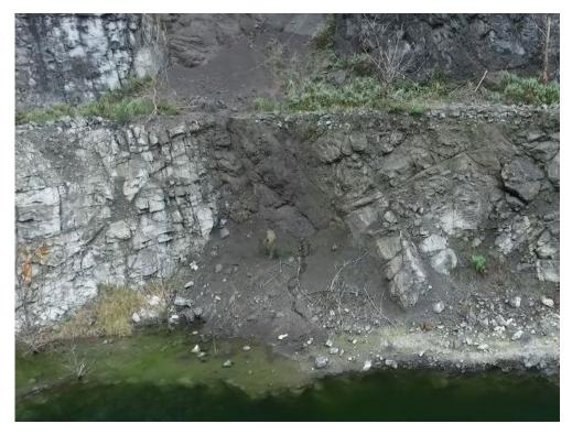
Plate 21. View of fractured rock and fragmented muddy breccia lowermost batter of the west wall.
