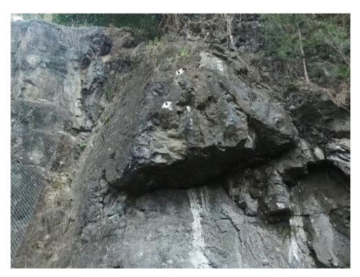
Plate 20. View of overhanging rock (muddy breccia) with rock bolts.
