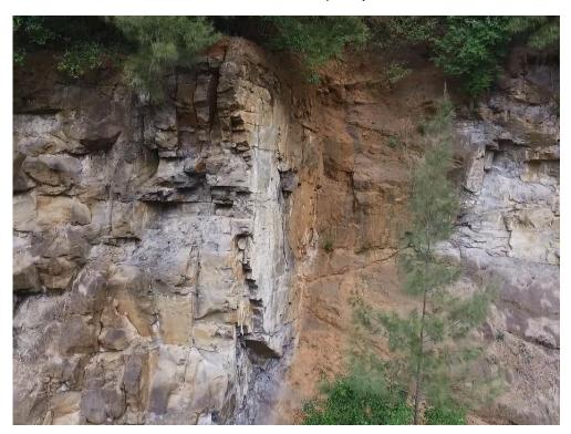
Plate 18. View of previous wedge failure and closely spaced joints on western area of south wall.
