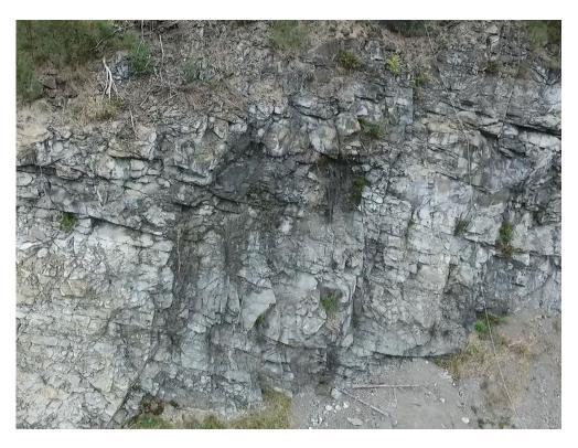
Plate 16. View of highly fractured, water stained batter below access road on south wall.
