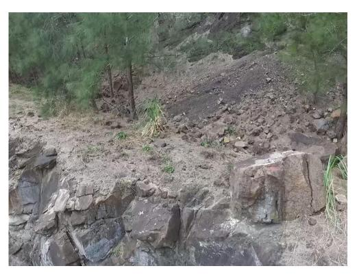
Plate 7. Rock debris accumulations on bench.
