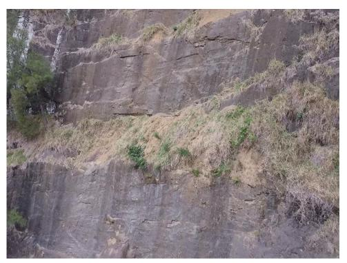
Plate 14. View of possible failure surface in muddy breccia on eastern south wall.
