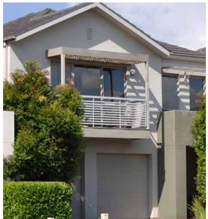
Figure 3.1(e): Sun shading devices are essential elements of a well designed home.(E)
