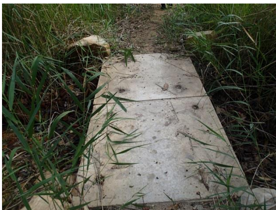
Figure 3.10: Culverts Allowing Catchment Inflows to the Wetland
