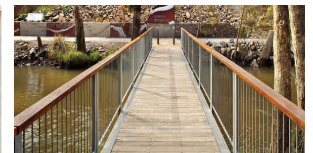
Timber Bridge (subject to future funding)
