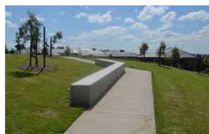
Concrete Footpaths & Walls
