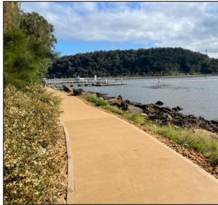
Coloured concrete footpath to tie in with existing foreshore path
