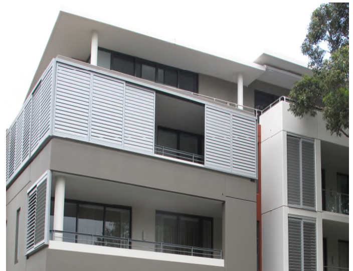
Figure 9.6-m: Balconies should incorporate operable louvres (E)
