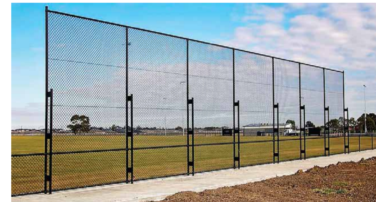
Ball stop net fencing, approximately 4m high located in front of new amenity building (suggestion only)
