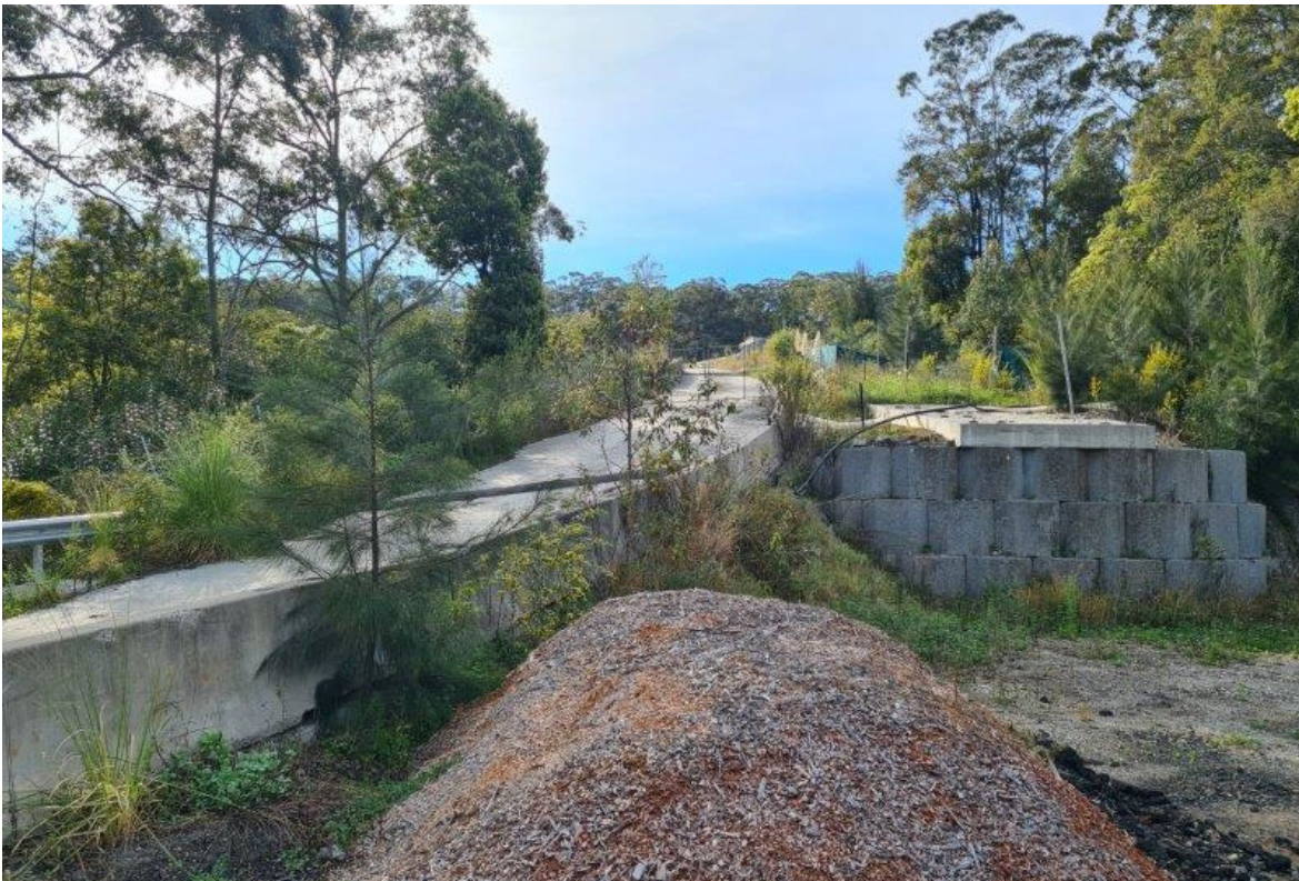
Photograph 7 Existing drainage pathway – under road
