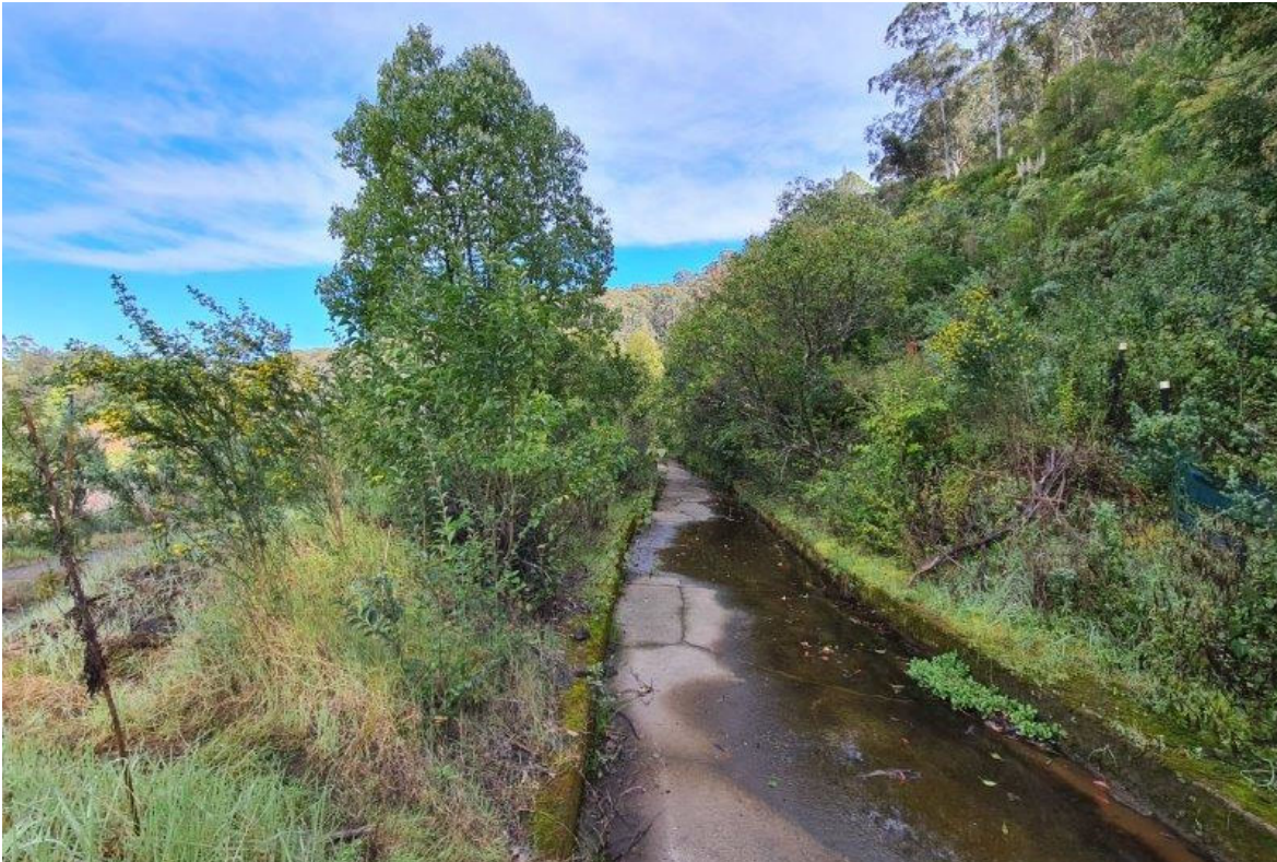
Photograph 10 Existing drainage pathway – concrete channel
