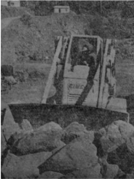
Figure 6. Work in Hornsby Quarry, 1961 (Source: Daily Telegraph, 24 March 2015)
