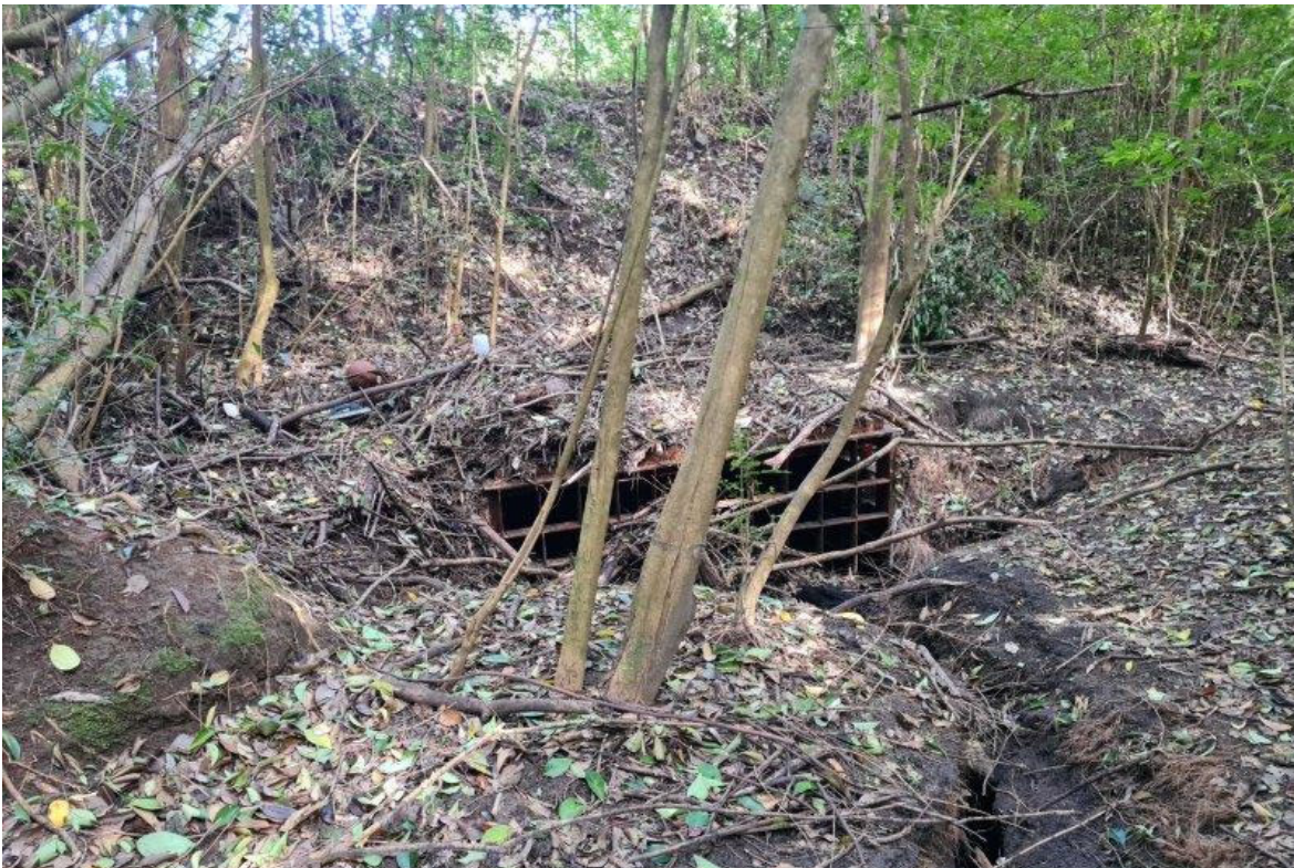
Photograph 9 Existing drainage pathway – pit/culvert
