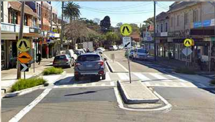
EXAMPLE OF RAISED PEDESTRIAN CROSSING
