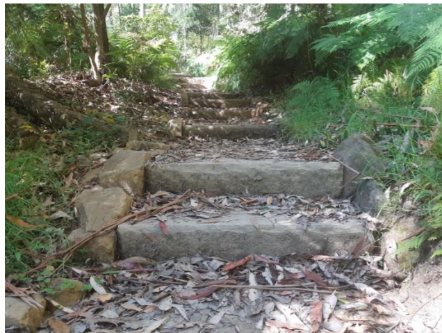
Example of sandstone steps to be installed.
