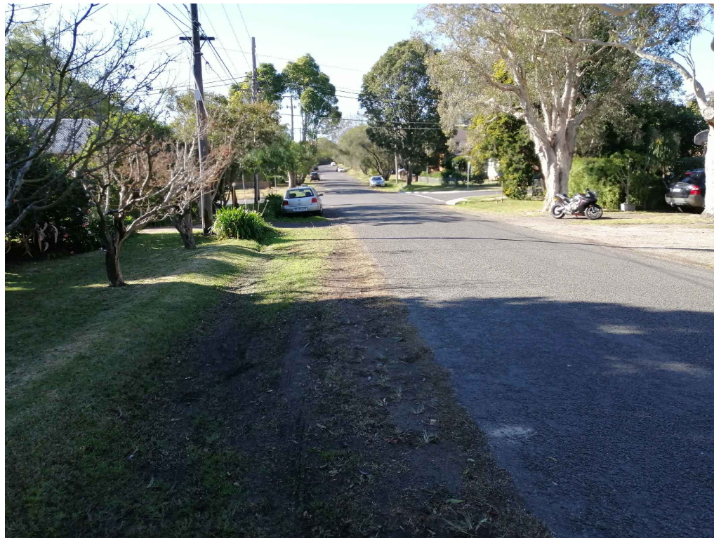
COLAH ROAD LOOKING EAST FROM OPPOSITE No.15
