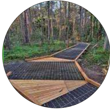
RAISED WALKWAY Fibre reinforced plastic decking with timber decking inserts
