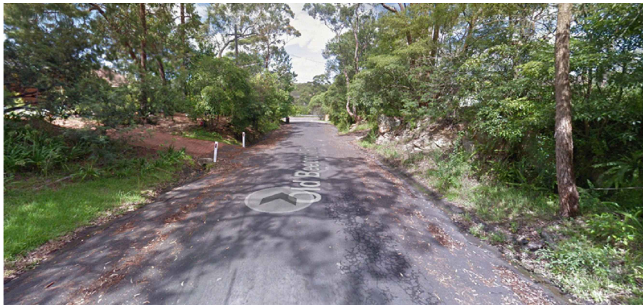
OLD BEECROFT ROAD LOOKING SOUTH FROM OPPOSITE No. 25
