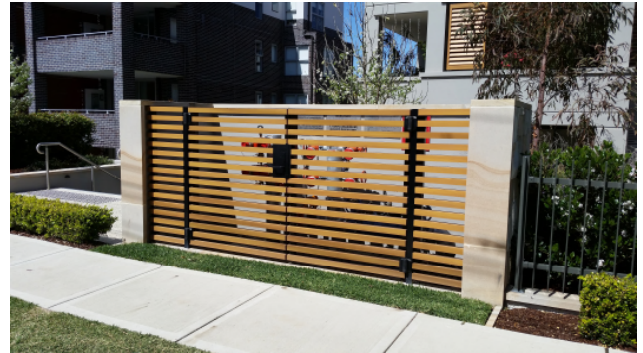
Figure 3.4-j : Example of the preferred style of screening for fire hydrants.
