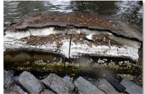
Polystyrene leaking from this pontoon in Cogra Bay
