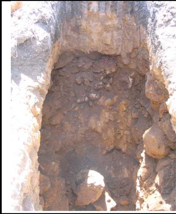
Photo of northern pit face; note the collapsing sidewalls.
