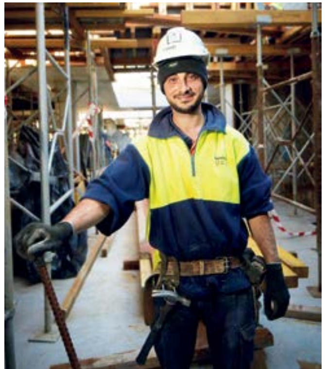
Working on Hornsby Aquatic Centre
