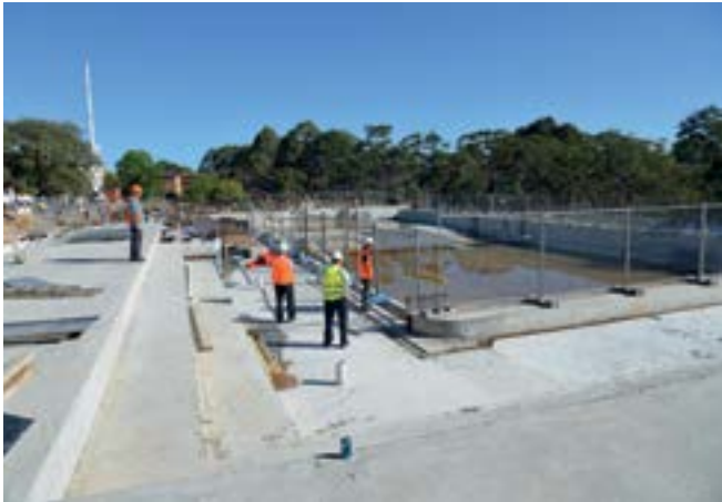
Hornsby Aquatic Centre construction has continued on schedule throughout the year
