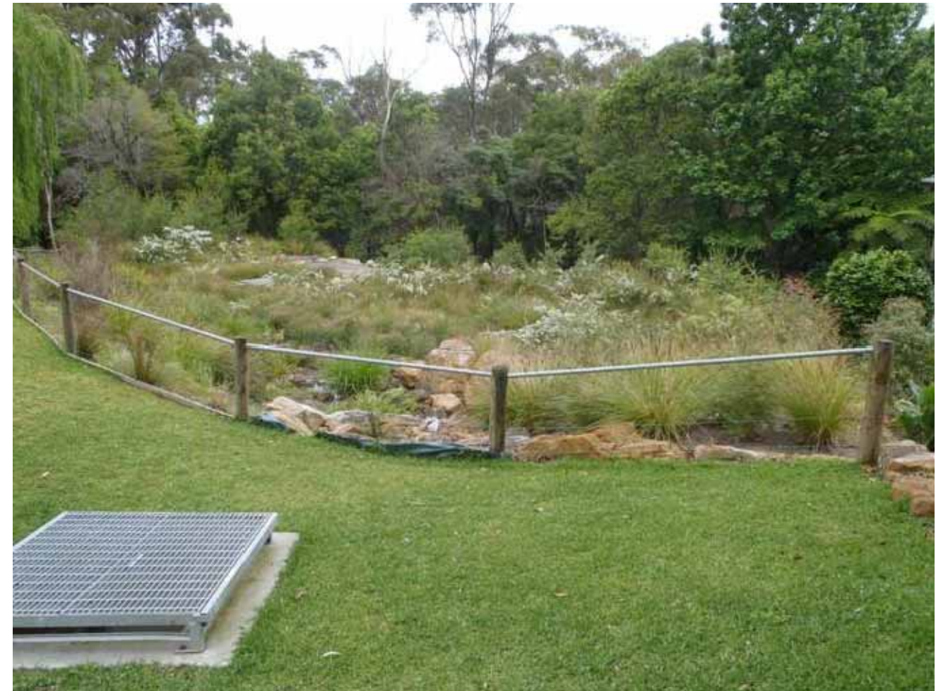
EXAMPLE OF COMPLETED BIO-FILTRATION & WATER HARVESTING BASIN
