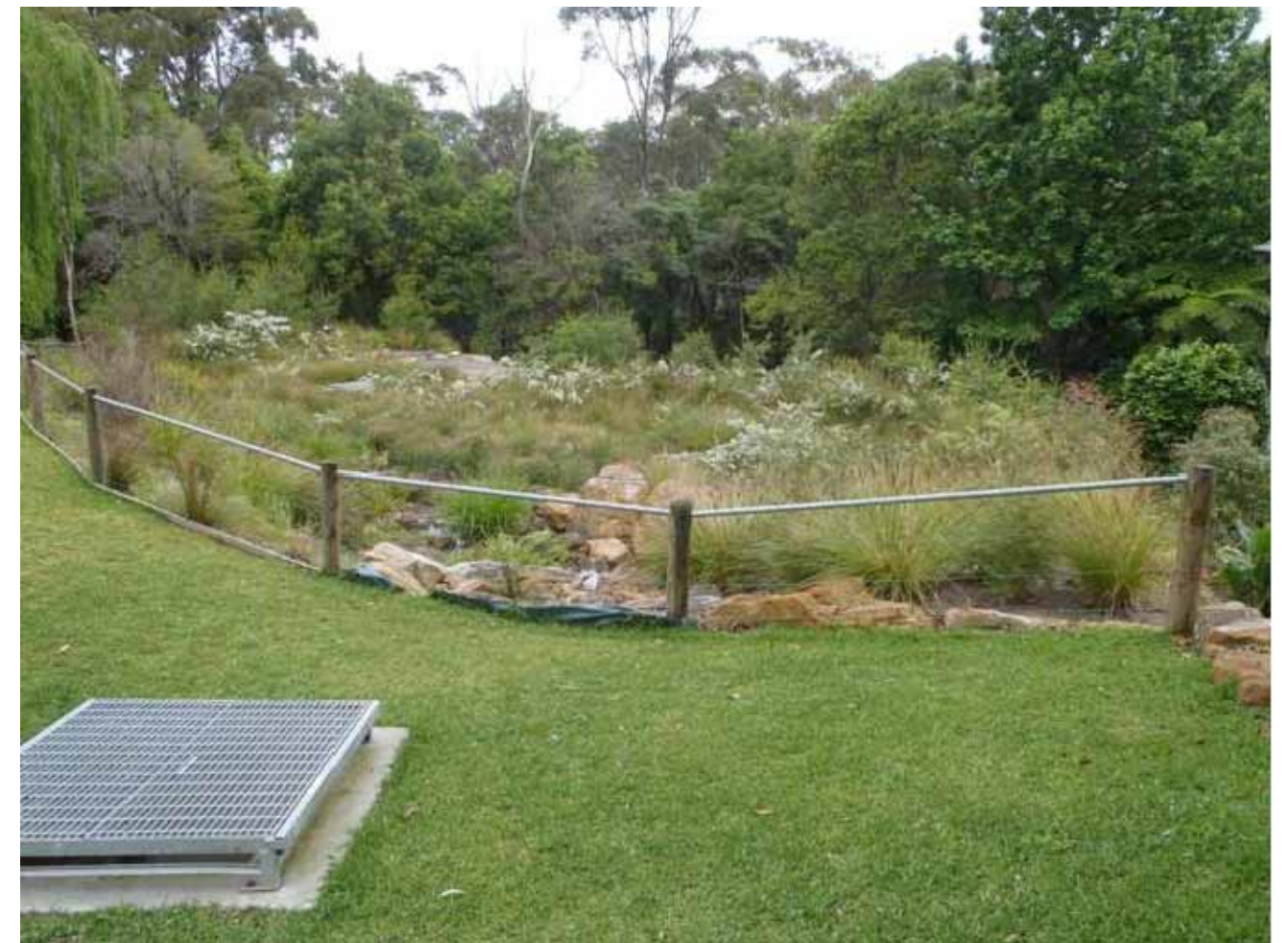
EXAMPLE OF COMPLETED BIO-FILTRATION & WATER HARVESTING BASIN
