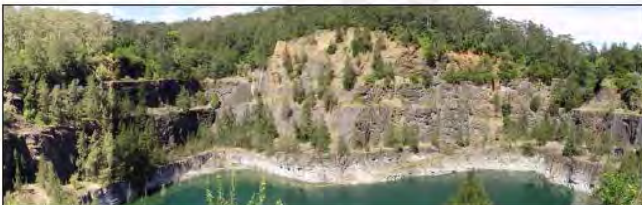
Hornsby Quarry - view from northern side of quarry, looking south showing fill areas
