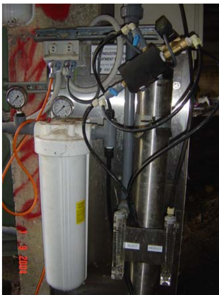
Figure 7 Reverse Osmosis (RO) Filtration Unit at Hornsby Pool.
