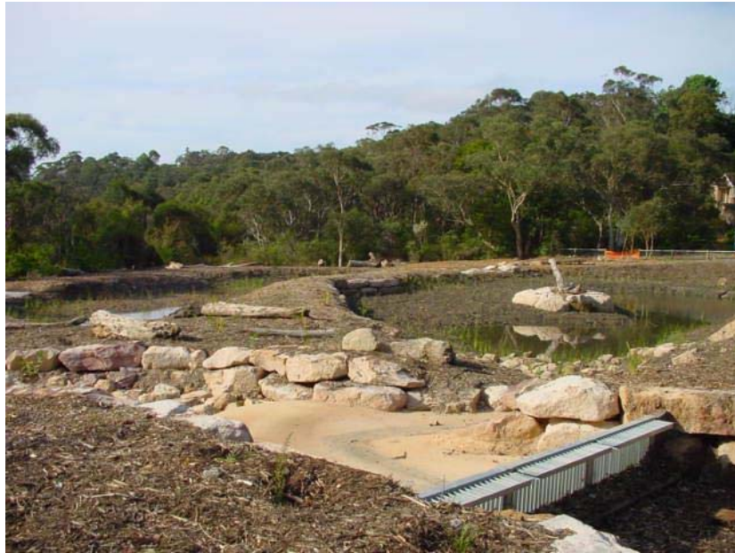
Figure 5 Clarinda Street wetland, Berowra
