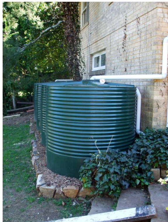
Rainwater tanks in Pennant Hills
