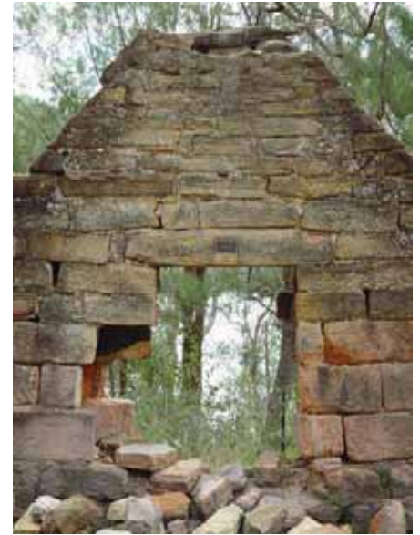
Photo 11. Remains of Church wall
