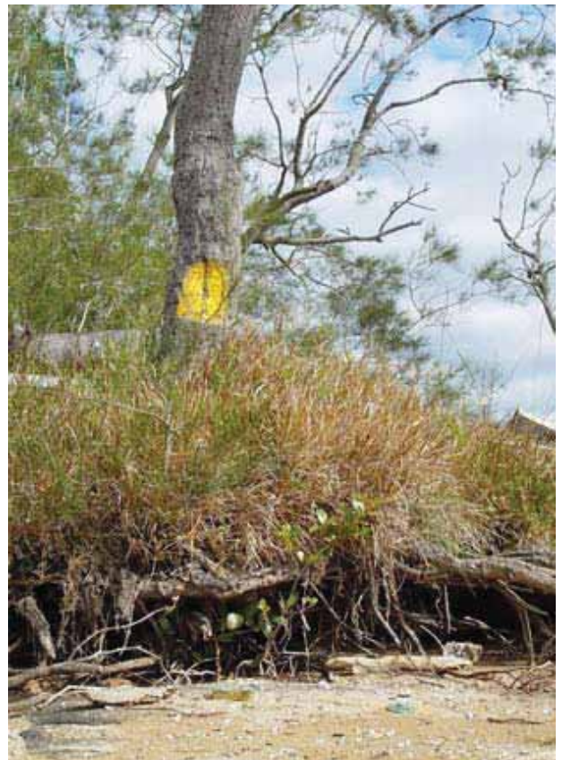
Photo 20. Foreshore erosion in the north-east corner of Bar Island - undercutting of the bank caused by wave action; the Casuarina glauca is important in strengthening the soil integrity
