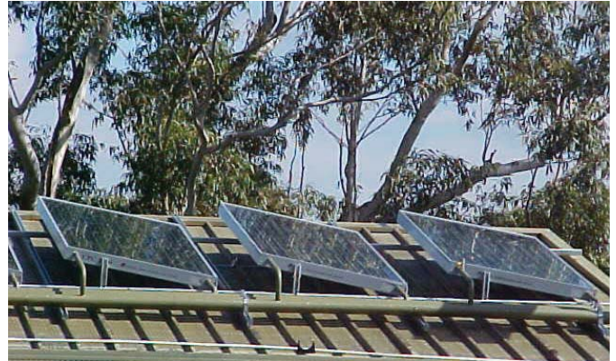
Solar collectors at Hornsby Aquatic Centre
