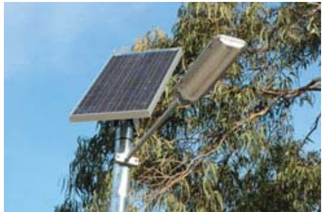
Solar street lights at Brickpitt Park, Thornleigh
