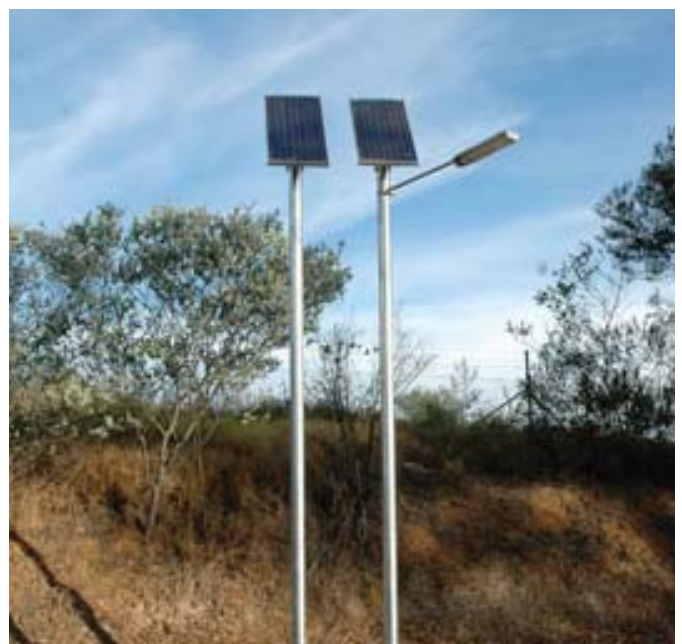
Solar street lights at Brickpitt Park, Thornleigh
