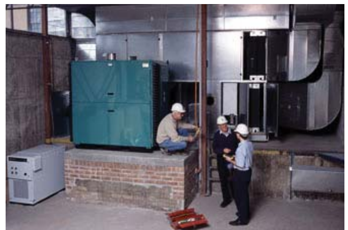
Construction of Cogeneration System at Hornsby Central Library
