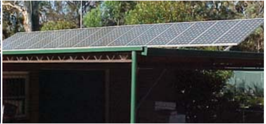
Solar panels on the Hornsby Community Nursery
