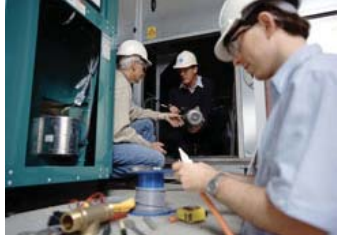
CSIRO installing the cogeneration system at Hornsby Central Library
