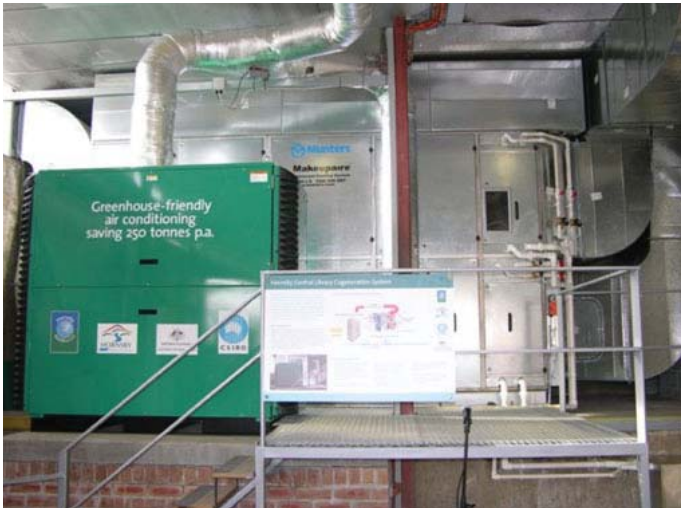
Cogeneration System (TrigenAir)
