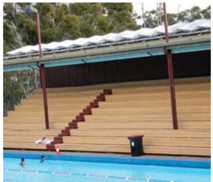
Solar collectors at Hornsby Aquatic Centre
