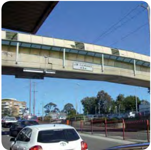
Hornsby pedestrian overbridge
