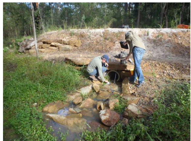
Plate 12 Water quality testing of harvested stormwater, Thornleigh Biofilter/stormwater harvesting system
