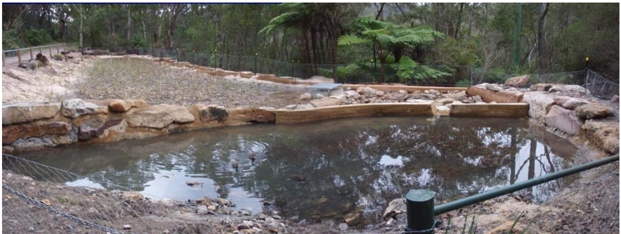
Plates 10-13: Pecan Place, Cherrybrook – Biofilter Works.
