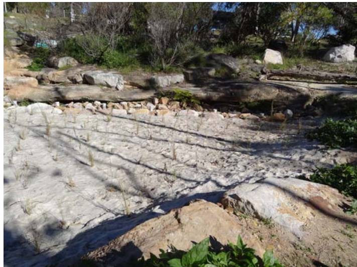
Plates 14-16: Biofilters completed in 2013-2014 Spedding Road, Hornsby Heights Appletree Drive, Cherrybrook (with graduated trash rack) Murralong Road, Mount Colah (retrofit of a sediment basin to biofilter)
