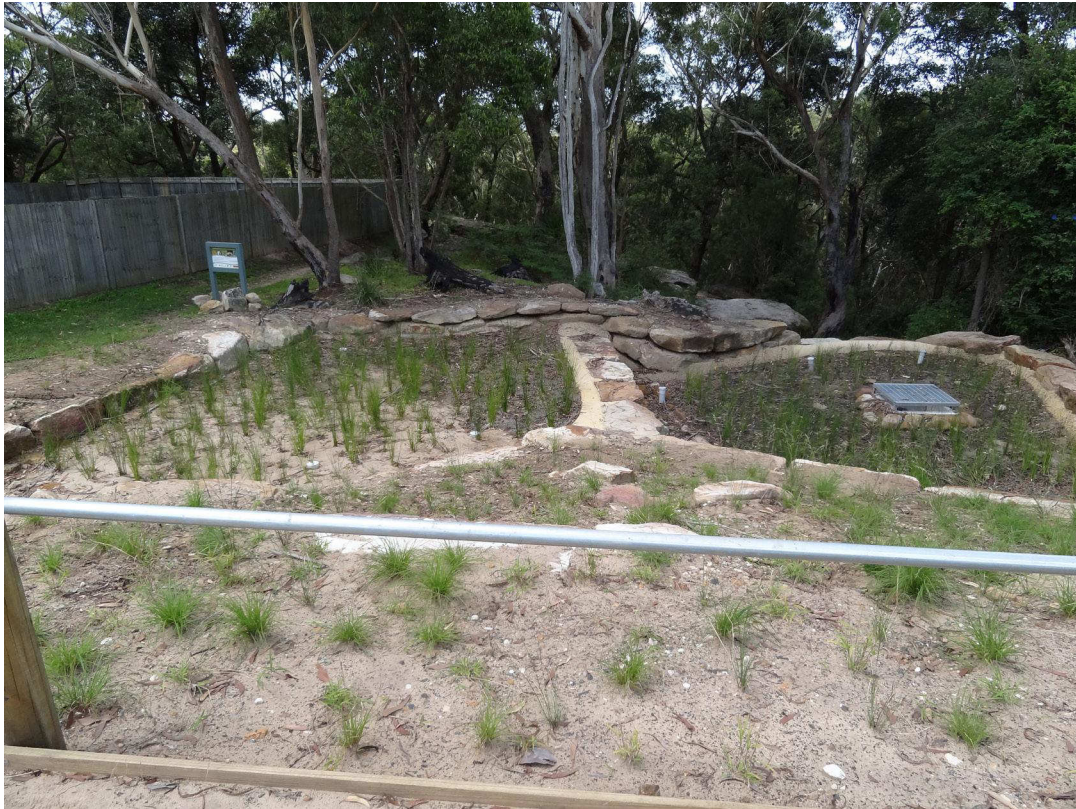
Plate 1 – Eastcote Road, North Epping – Bioretention System
