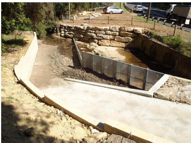
Plates 8-11 – Flametree Crescent, Cherrybrook – Trash Racks
