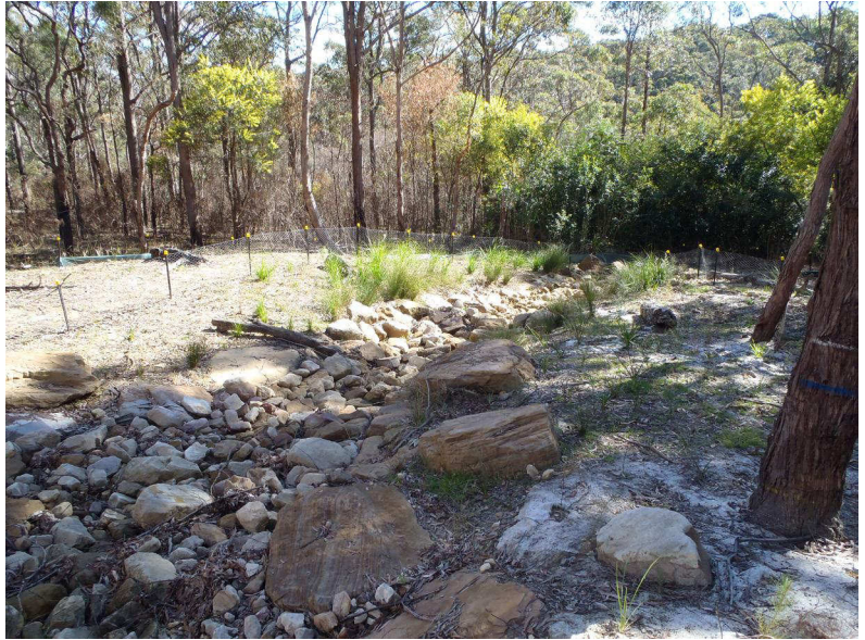
Plates 11-12 – Essex Street, Epping, Lawson Road, Cherrybrook - Drainage line rock armouring
