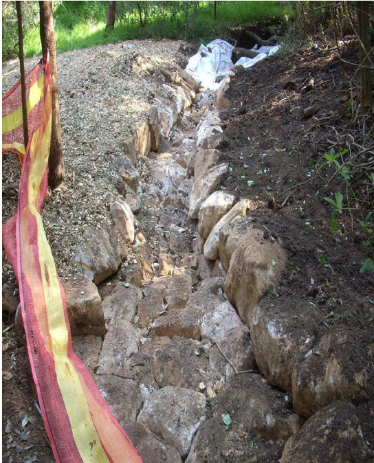
Plates 11-12 – Essex Street, Epping, Lawson Road, Cherrybrook - Drainage line rock armouring
