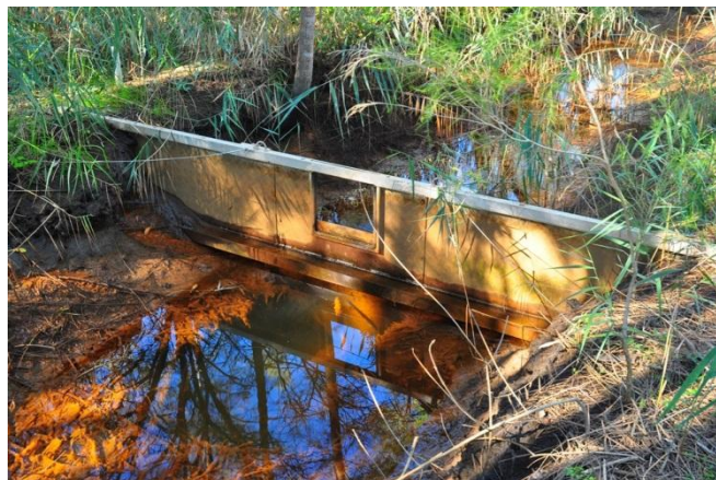
Figure 12 Existing Tidal Weir Control and Associated Scour Pool
